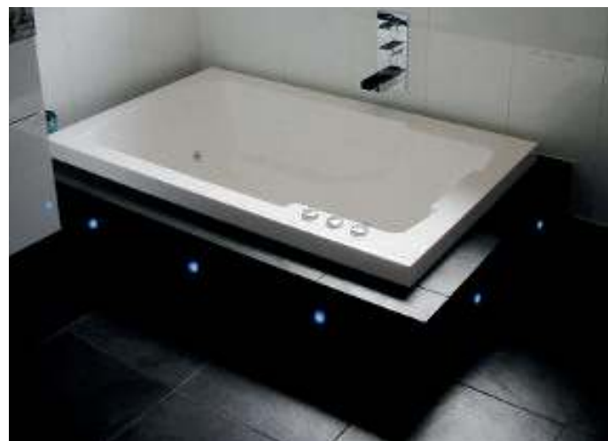
A Cabuchon tub, partially sunken into a floor, inset above a tiled deck.
